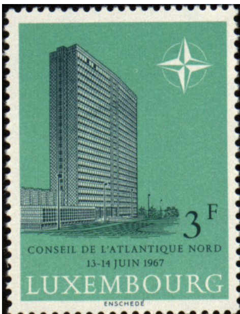
Tower Building (1967 stamp).
