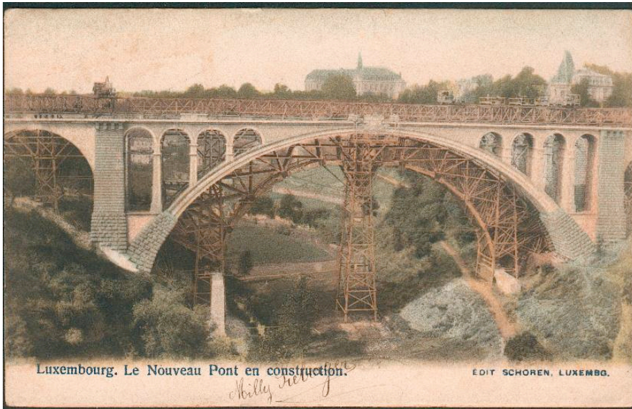
1902 postcard showing the Adolphe Bridge under construction.
