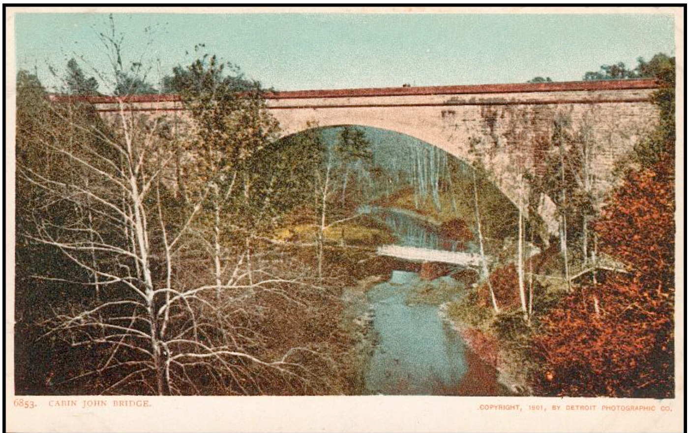
The Cabin John Bridge near Washington, D.C. — when it was completed in 1863, its stone arch was the longest of any bridge in the world (1903 postcard). This record held until the completion of the Adolphe Bridge 40 years later. The arch spans 220 ft., 59 ft. shorter than the central arch of the Adolphe Bridge.
