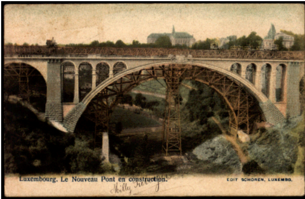
The Adolphe Bridge under construction (1903).
